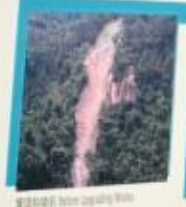
實施綠化工程前 Before Greening Works
